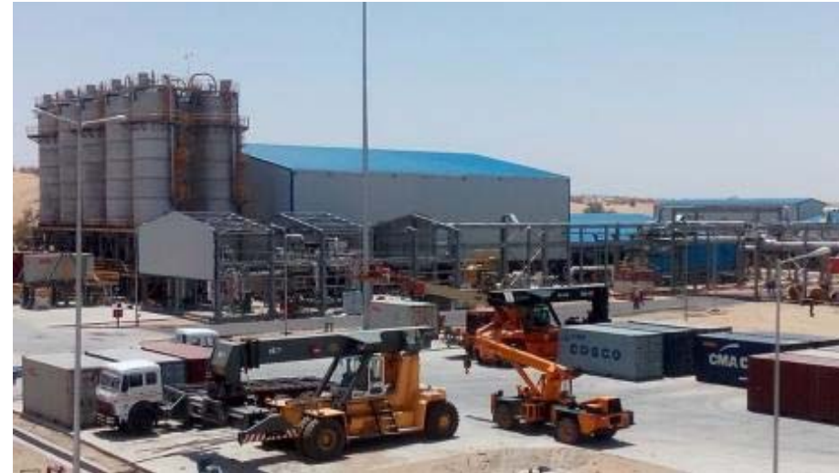
Central Polymer Facility, Rajasthan
